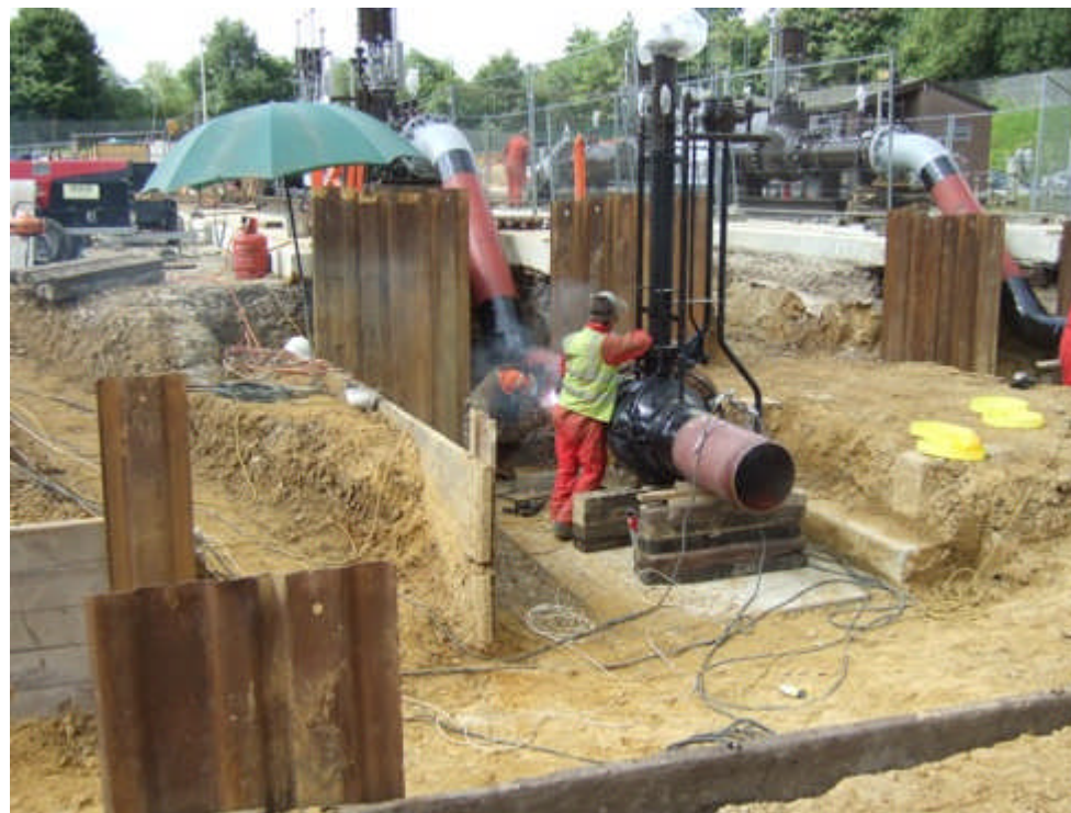
Pictured above: Welding of 18" diameter pipework at Braishfield AGI near Romsey 2009
